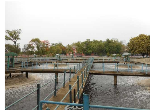
Existing Sewerage Treatment Plant to be rehabilitated
