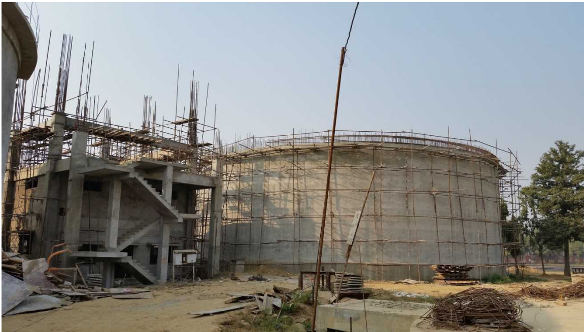
140 MLD New Sewage Treatment Plant under construction in Dinapur, Varanasi
