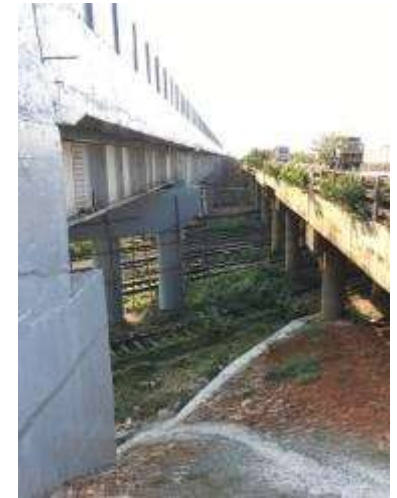
Access Road to Kamarajar Port (Ennore Port) (Left: New Road, Right: Old Road)
