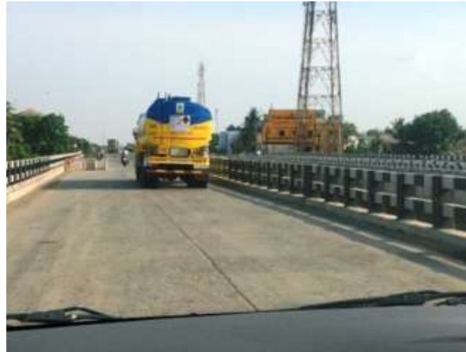
Access Road to Kamarajar Port (Ennore Port) Supported under TNIPP
