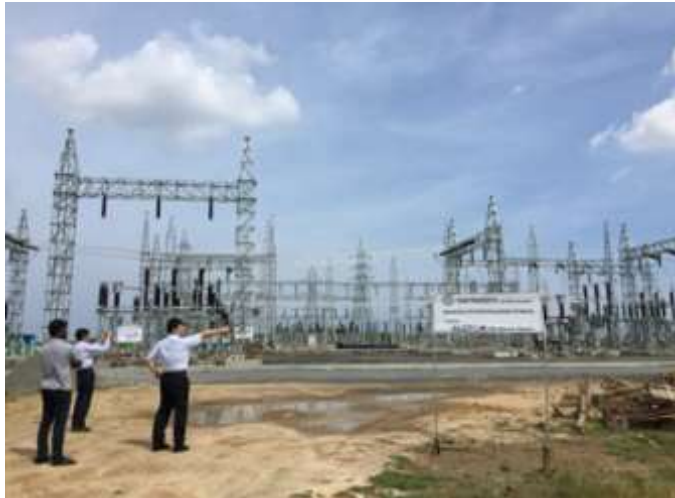
Substation at One Hub Chennai Industrial Park Supported under TNIPP
