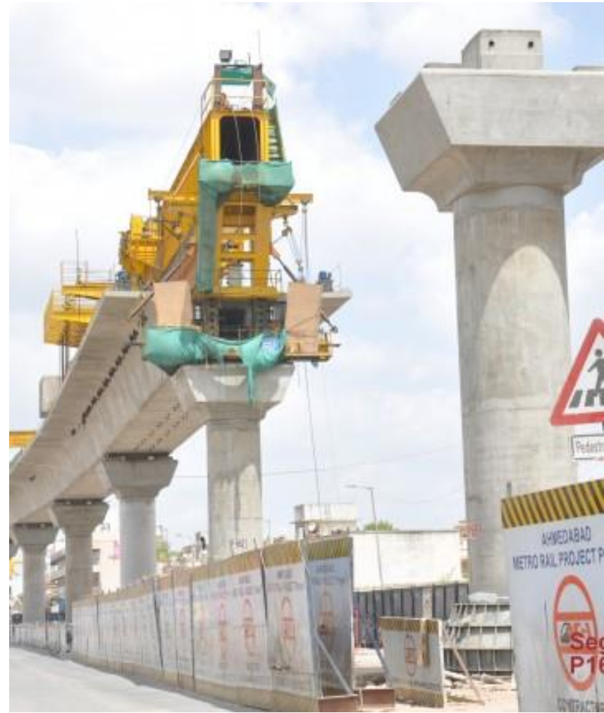
(Photo: Construction of Viaduct, JICA)
