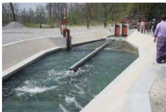
Rehabilitated irrigation system
