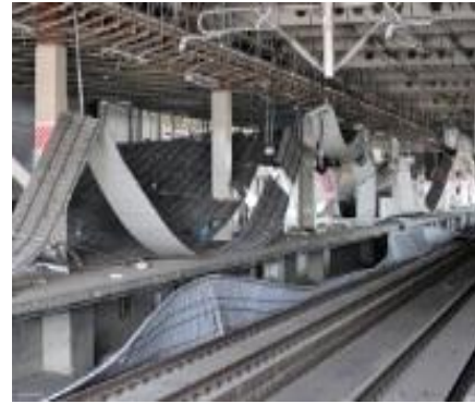
Collapsed roofs of Sendai station
