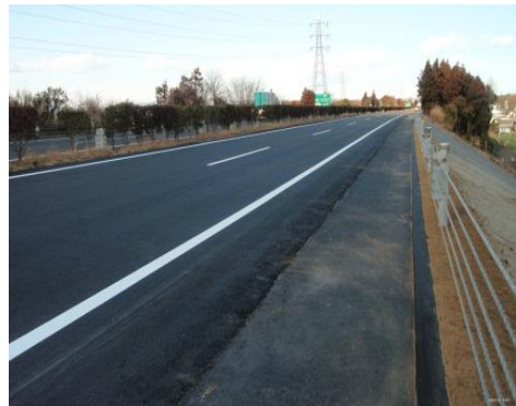
Restored Joban Expressway (March 17, 2011)
