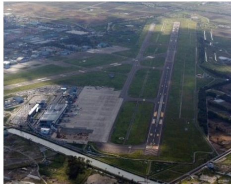
Restored runways of Sendai Airport (April 2011)
