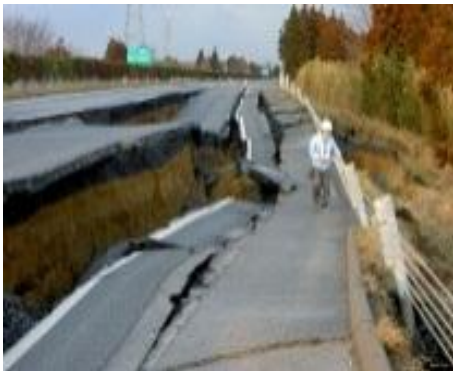
Subsided Joban Expressway
