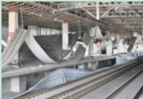
Collapsed roofs of Sendai station
